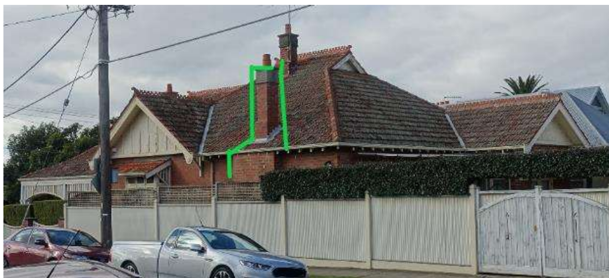
Figure 35. View of the east side and rear of 17 Park Street. The new chimney and chimney breast are indicated, as well as the approximate line separating the original house (left) and 1990s extension (right).
