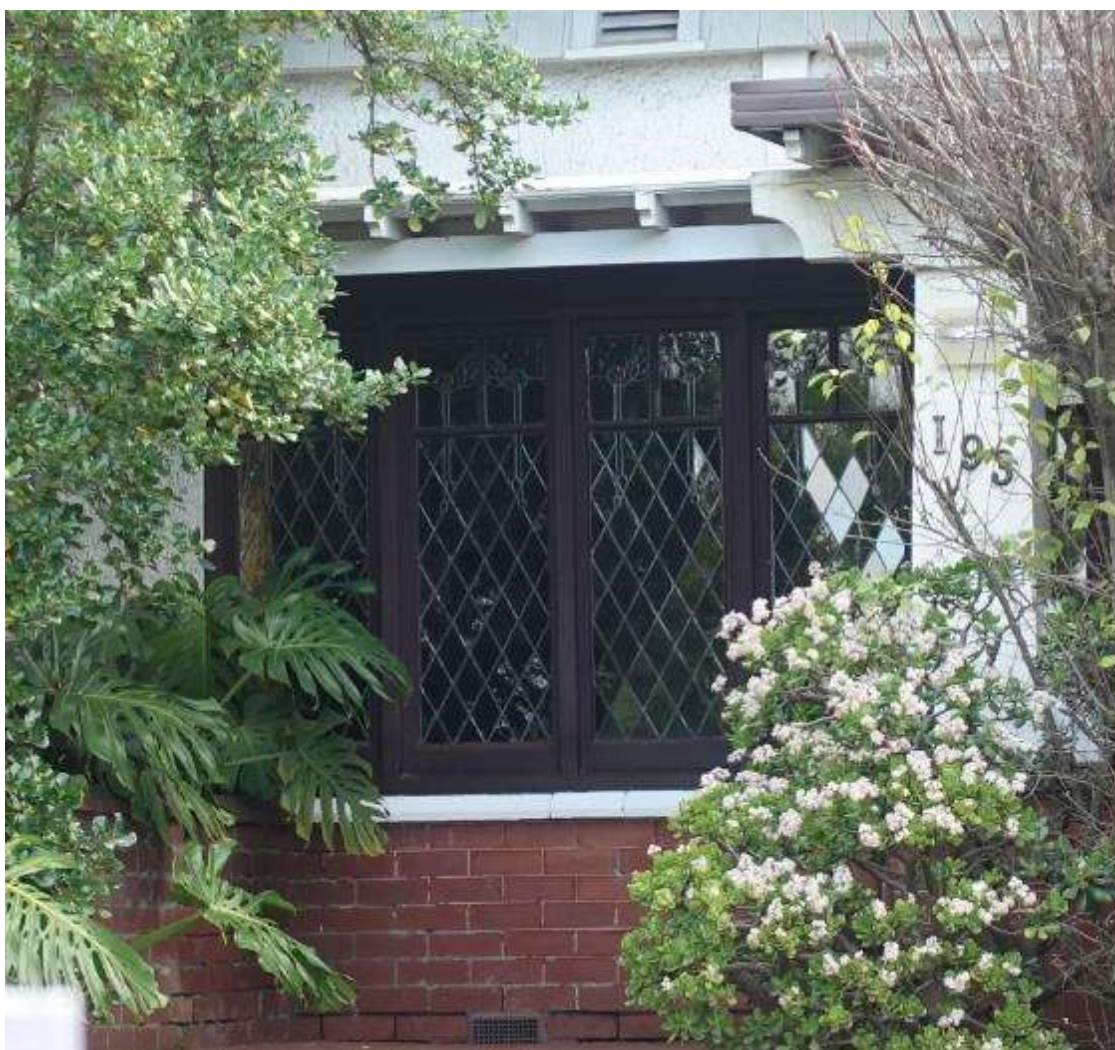
Figure 26. Leadlight windows of the front façade. Matching joinery details to the bay window hood and the front porch are also visible.
