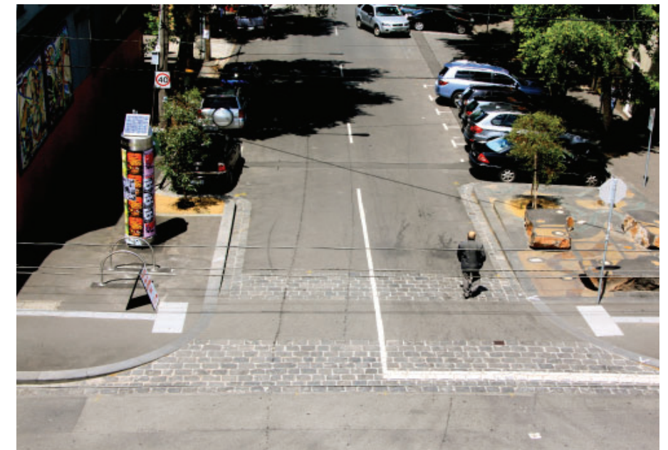
▲ Pedestrian crossing example with bluestone pitcher ramps to slow traffic. Consistent surface material and treatment is proposed for both raised and flat crossing arrangements.
