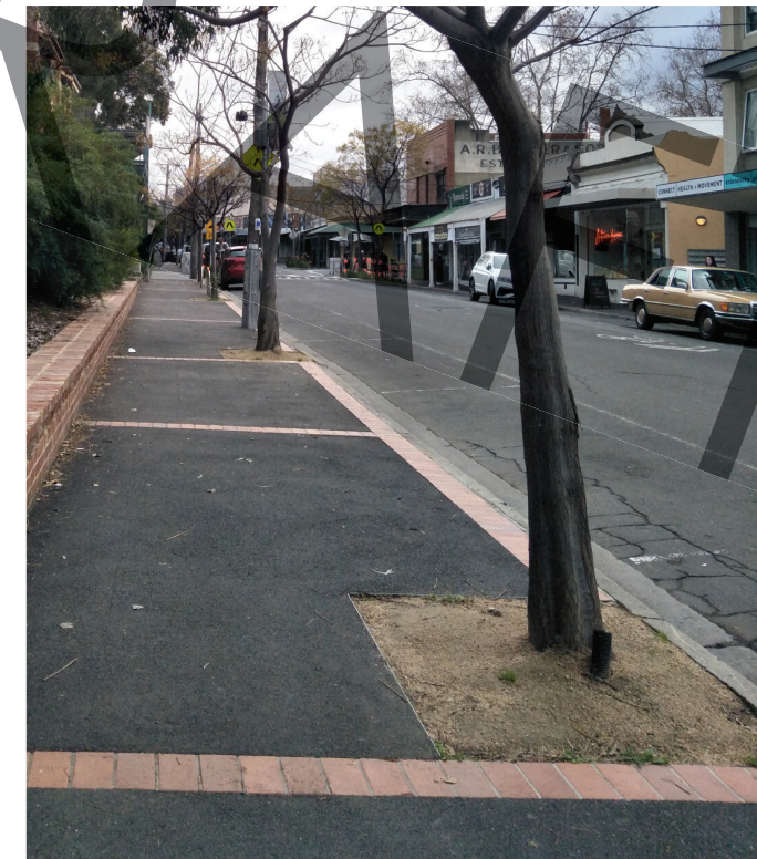
▲ Treepit in asphalt with steel edge
