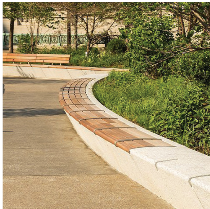
▲ Example of custom concrete seat/wall with timber inserts
